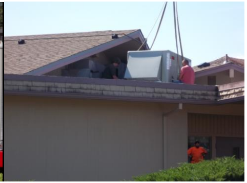
New unit in place
