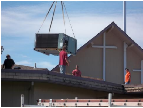
Old unit removed
