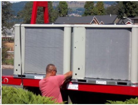
New unit on truck
