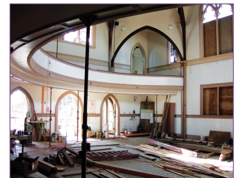
Kaumakapili under restoration 2003
