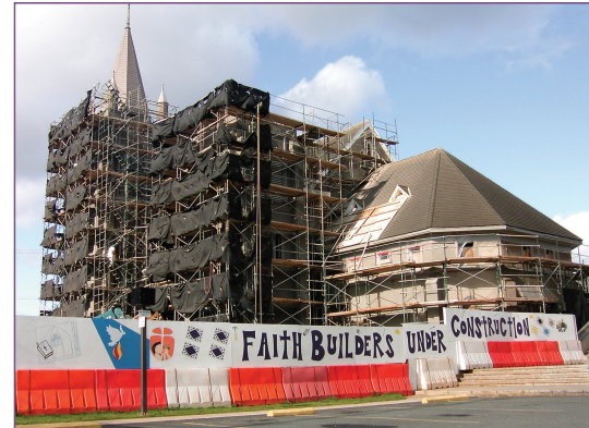
Kaumakapili under restoration 2003
