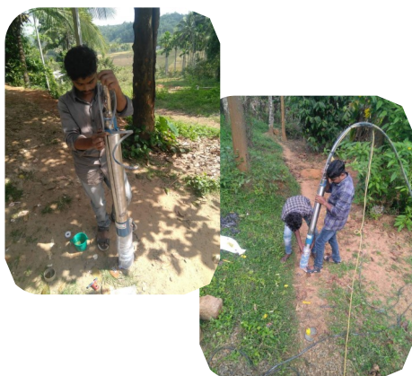
A new well being drilled
