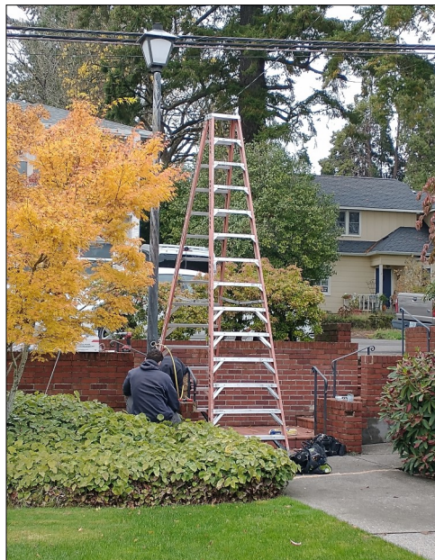
Upgraded LED lamp post lights with independent sensors and AC outlets.
