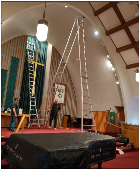
Brighter and more efficient LED lights installed throughout the chancel and sanctuary.
