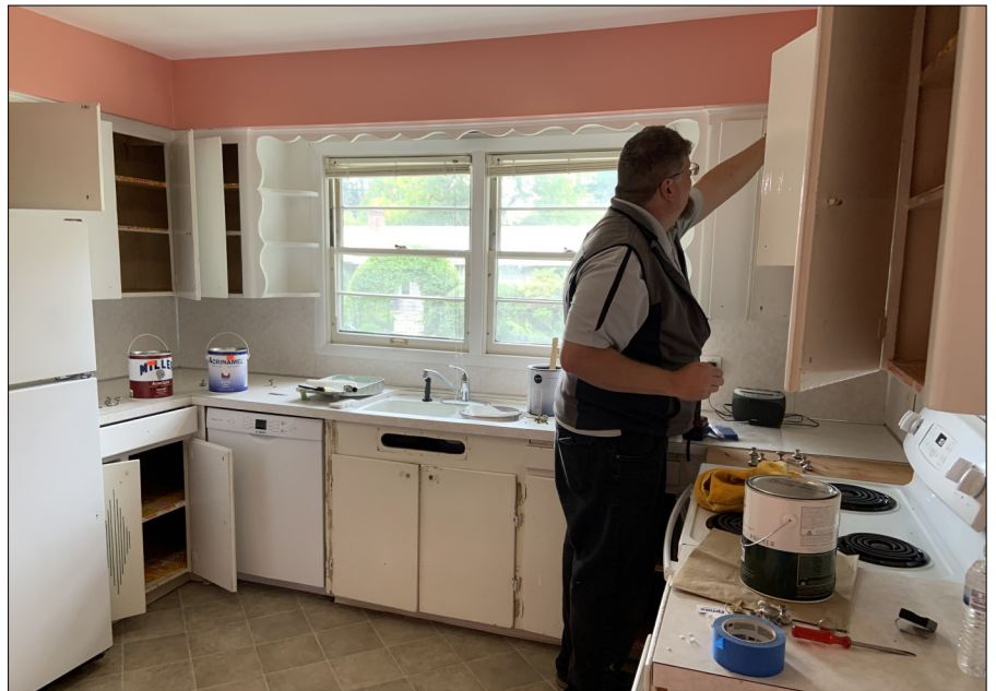
Gary Moen made necessary repairs and helped paint the Mission House.
