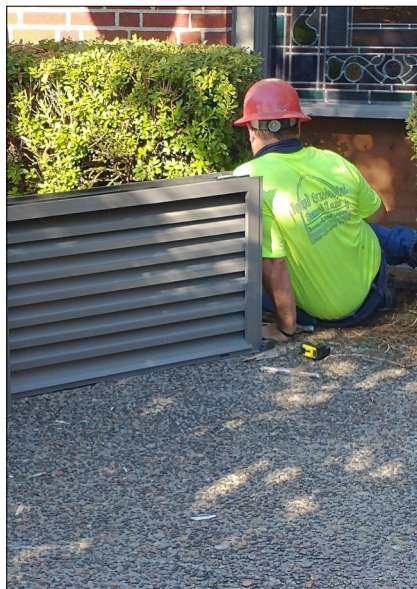
Above and below: New matching aluminum Louvers were installed.
