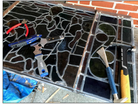
Above and right: It was discovered that this transept window was originally installed backwards. It was removed, disassembled, soldered together correctly, and reinstalled.
