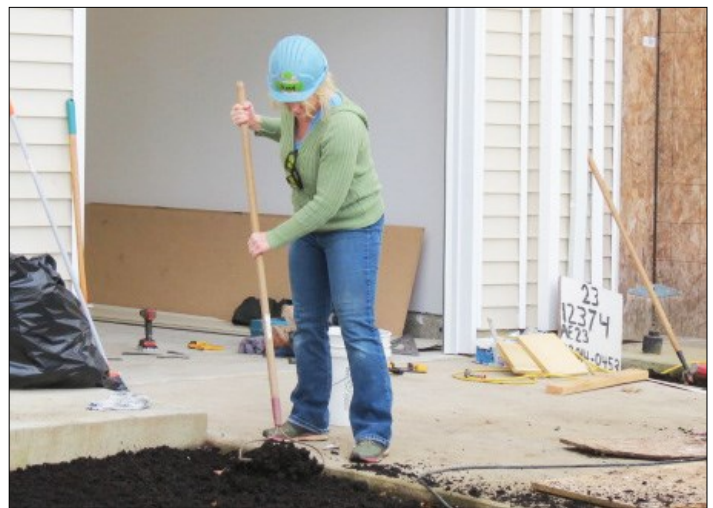
Valley member, Amy Rheingans, moving soil at the Allen Estates work site.
