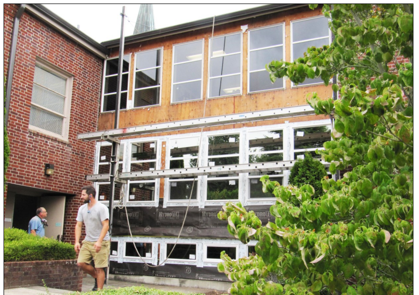
Above and right: New windows and siding are being installed on the south side of the church.
