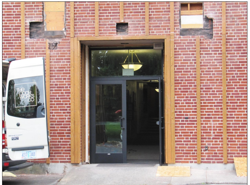
Right: New automatic doors have been installed in the East entrance. Boards are placed in front of the brickwork in anticipation of new siding and awning.
