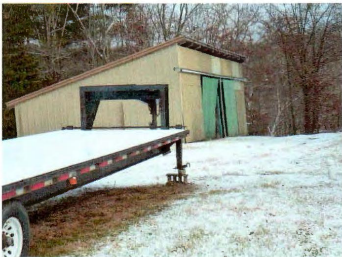
Open Pole Shed
