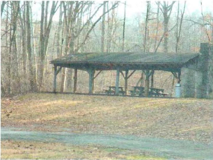
Shelter House at Picnic Area
