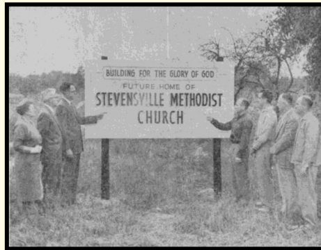
c. 1959 Building site for future home of Stevensville United Methodist Church on Ridge Road, Stevensville, MI Rev. Strohl was pastor at this time.
