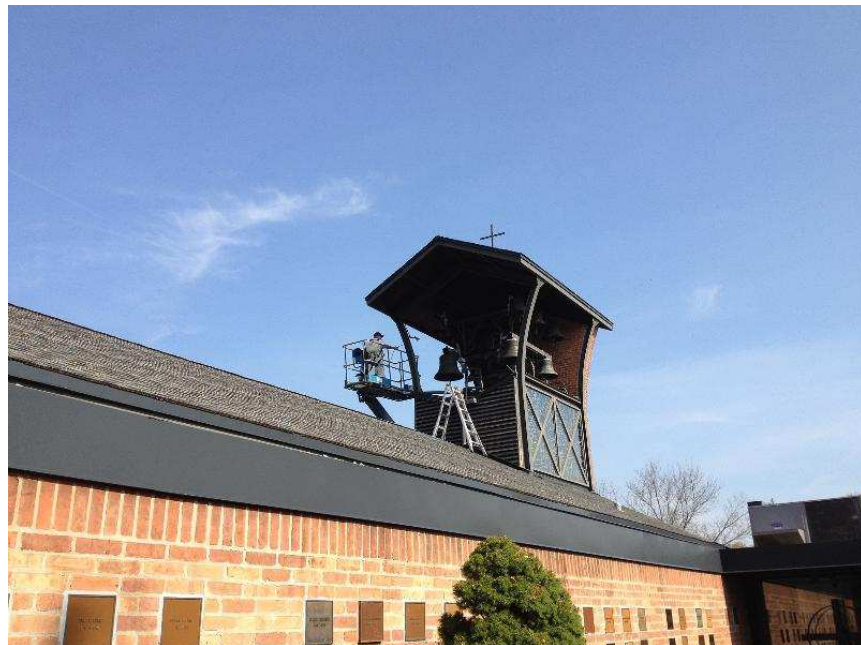
Painting the Bell Tower.
