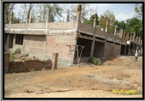
Mandla Clinic Construction
