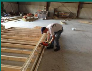
Mark Haines putting together a wall.
