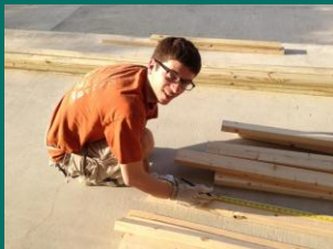
Justin Stevenson marking the boards to be cut.
