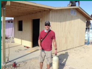
Gil spraying each of the houses for termites.
