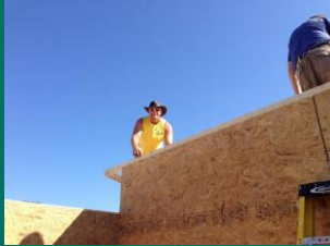
Jason working on the roof at one of the houses.
