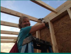
Lori also putting in hurricane clips.
