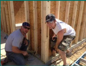
Steve and Cullen working to secure the house to the concrete.
