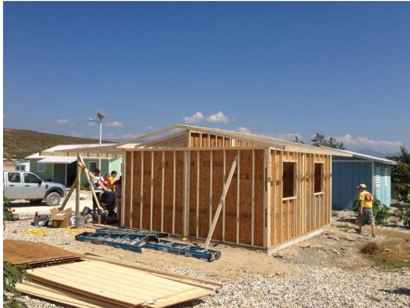
One of the three houses that the team worked on putting together, on Tuesday.
