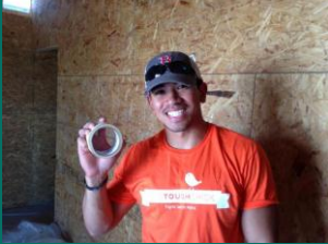
Frank getting ready to tape before they can paint the trim.
