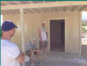
Justin S. and Mike ready to paint.
