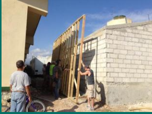
Some of the team getting the roof panels in place.
