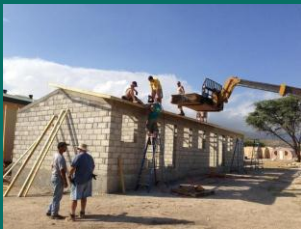
The team is securing the panels.
